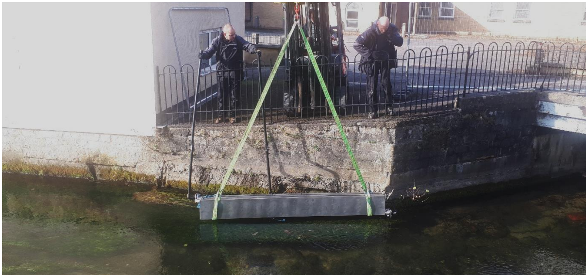
Figure 4: 3 panel FireFlo assembly being lowered into the watercourse
