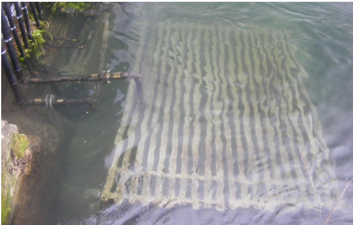
Figure 2: vertical bed mounted FireFlo panels (centre) alongside wall mounted panels (left)
