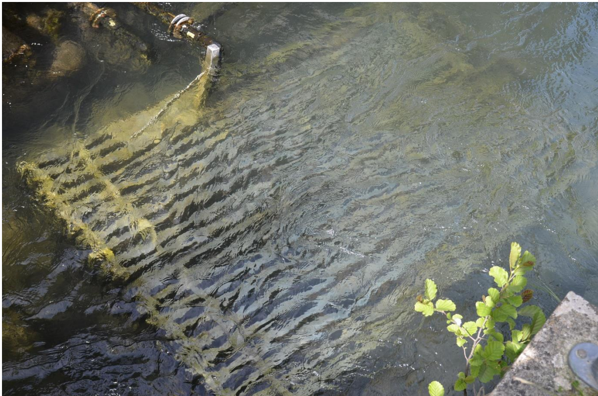
Figure 5: 20 off bed-mounted vertical FireFlo heat collectors after one year of operation
